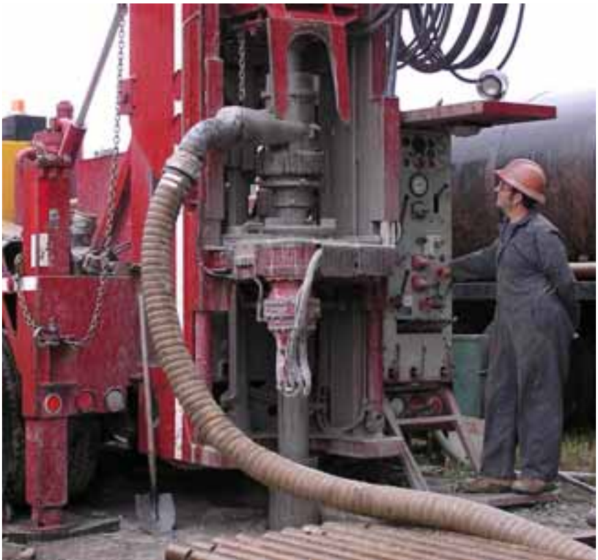
Figure 4.2 Installing a Groundwater-Monitoring well.
